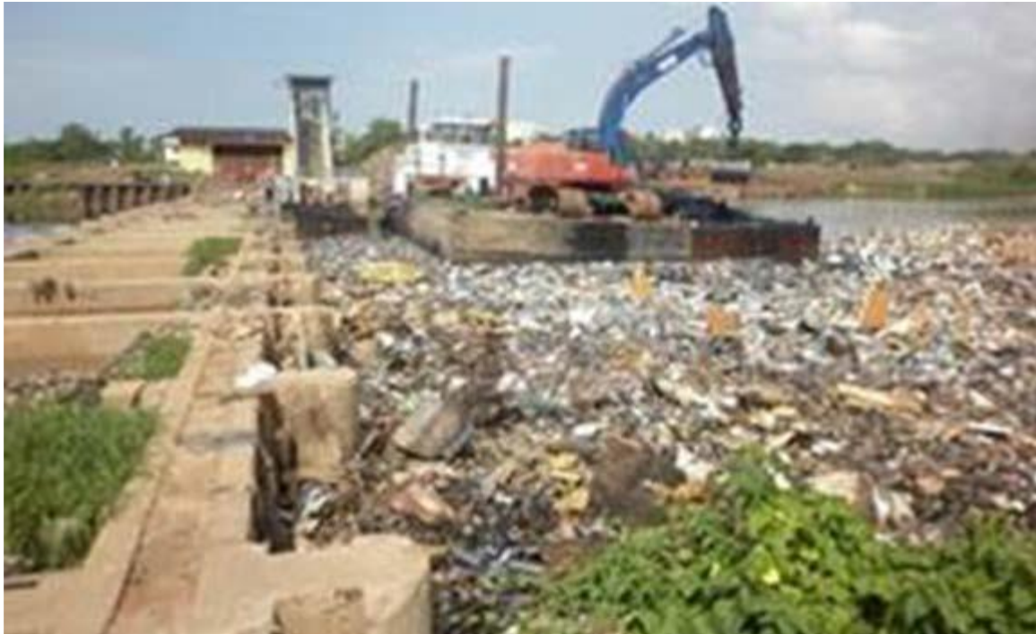
Fig.4: Photo of the Korle Lagoon Interceptor Weir
