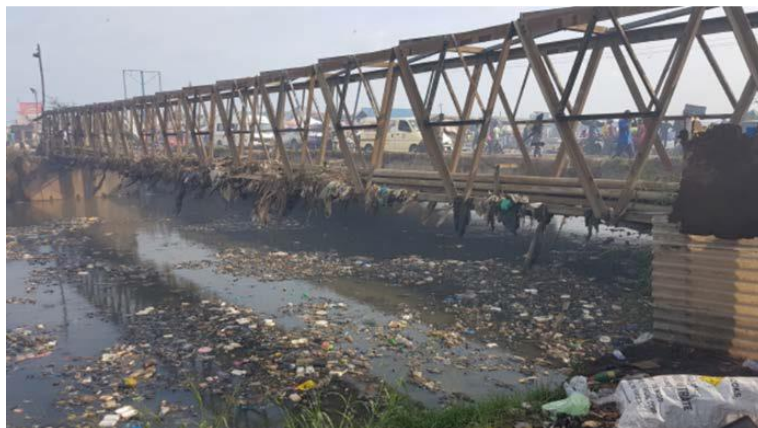
Fig. 7: Abossey Okai Bridge
