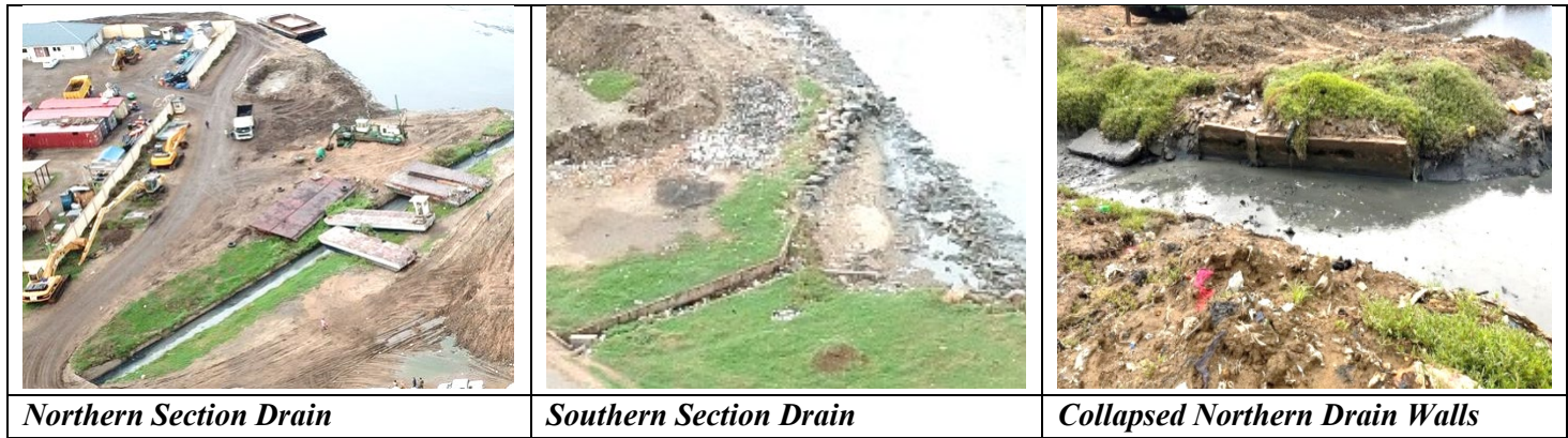
Figure 5.6 Drainage Channel at the Korle-na Site
