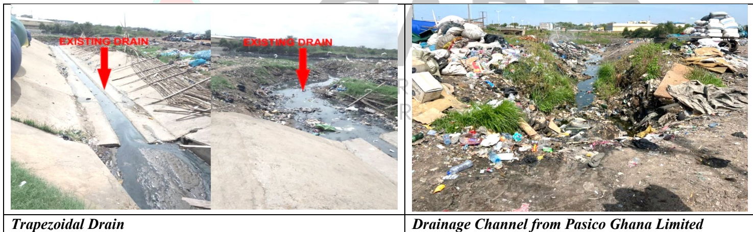
Figure 5.7 Existing Drainage Channel at the Pasico Site
