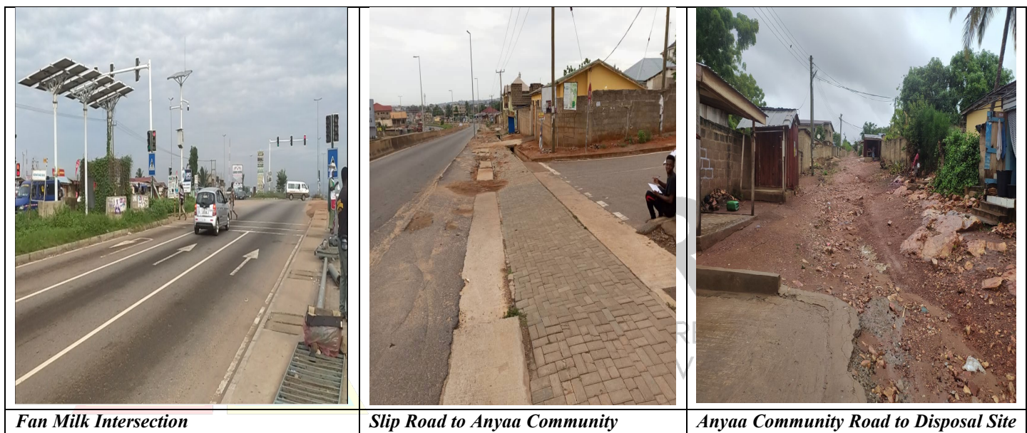
Figure 5. 21 Access Route to Anyaa Disposal Site
