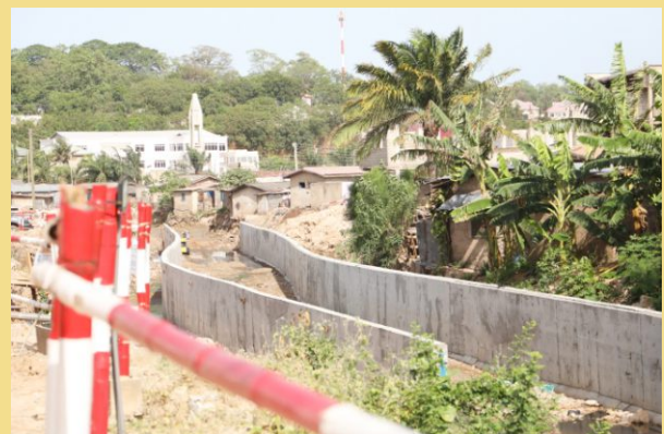
Community upgrading works in Alogboshie
