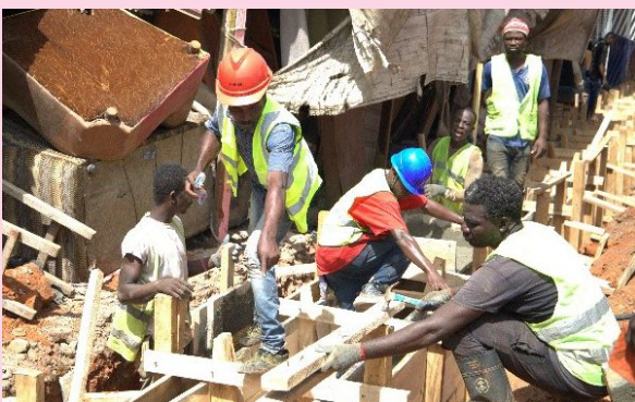
Community upgrading works in Nima
