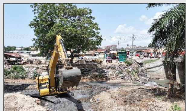
Community upgrading works in Akweteyman
