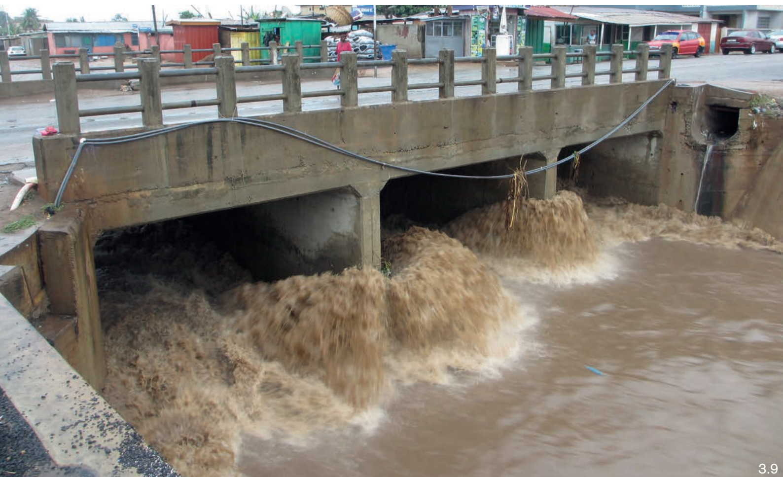
Figure 3.9: Heavy drainage due to insufficient capacity of drains
