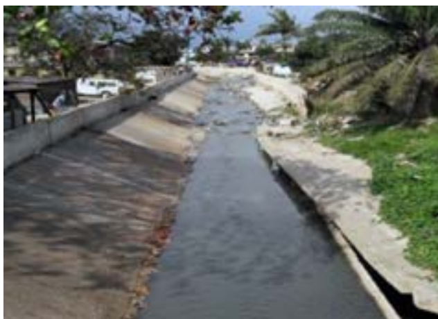
b. Collapsed walls of the Nima Drain
